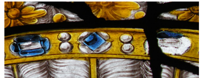
Failing blue enamel - Hamsterley Hall
